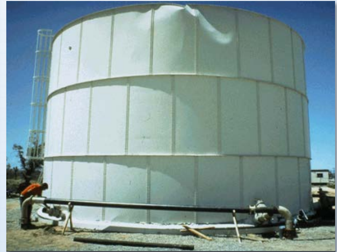
Example of Potential Seismic Damage
