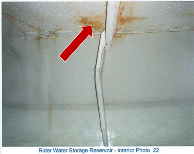
Tank Interior Corrosion (Four Steel Tanks)
