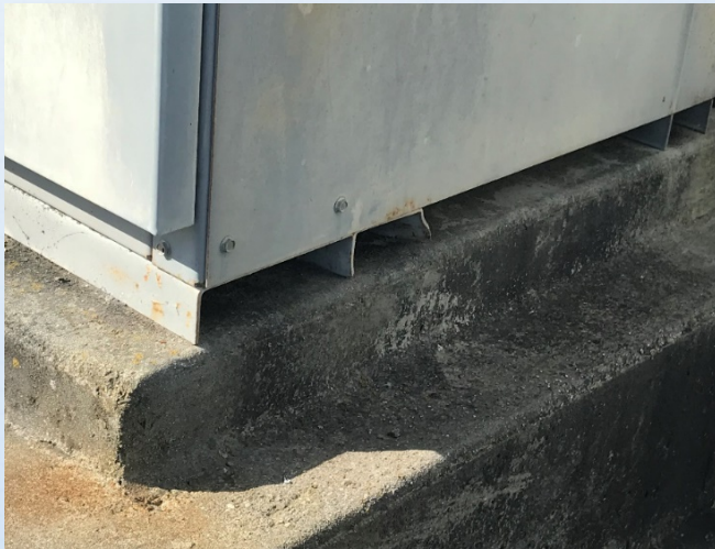
Electrical Panel Seismic Anchors
