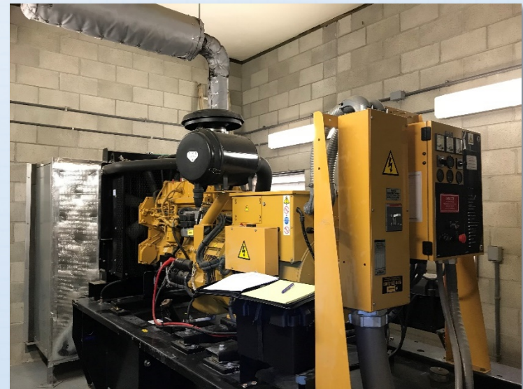
New emergency generators at Wells 14 & 18
