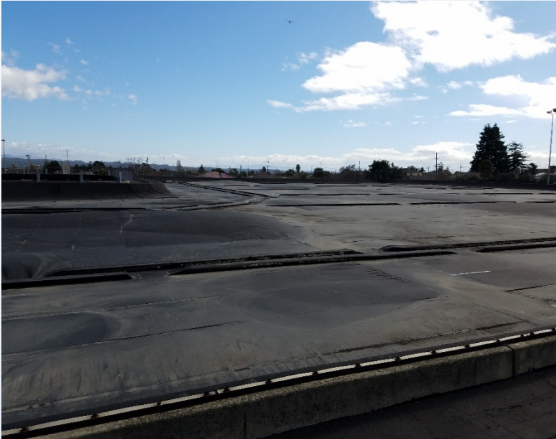
Freedom Reservoirs with Floating Covers (0.7 and 5.3 MG)
