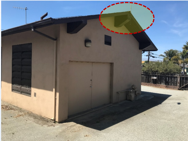
Anchorage of Roof Beams to Walls
