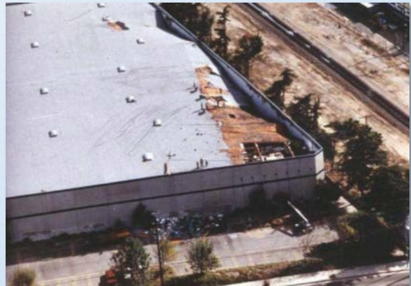
Example of Roof Collapse
