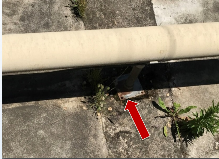
Replace Anchor Bolts at Pipe Supports
