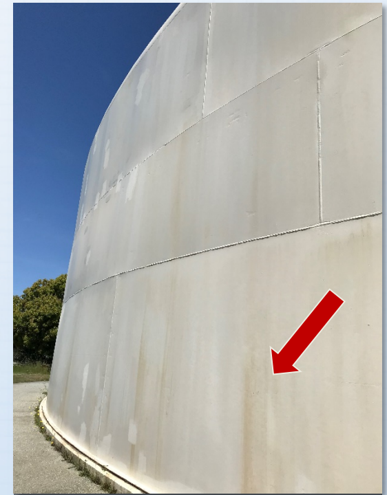
Tank Exterior Corrosion (Airport Tank)
