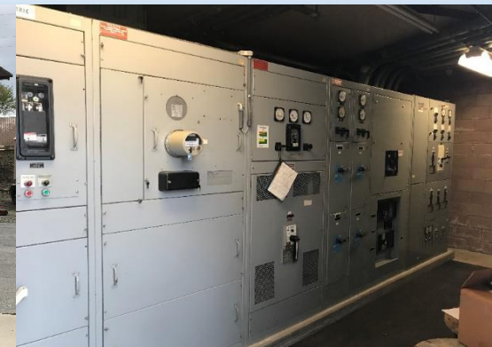
Main Switchgear Building and PG&E Transformer
