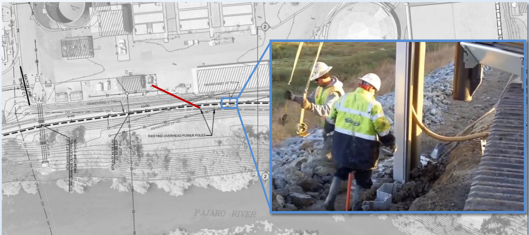
PG&E Service Entrance Affected by Proposed Sheet Piles
