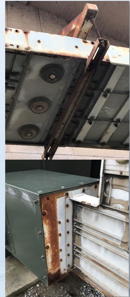
Significant Corrosion (Transformer Busway)
