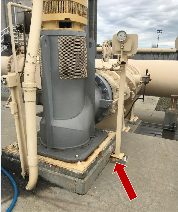
Replace Anchor Bolts and Grout (Recycle PS)
