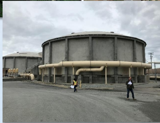
Trickling Filters
