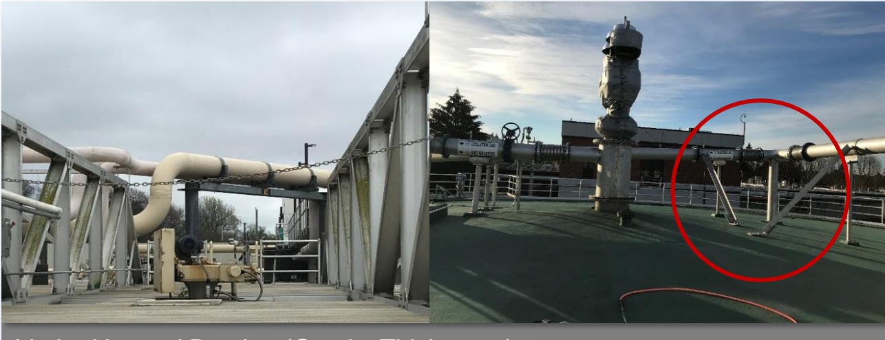
Limited Lateral Bracing (Gravity Thickeners)
