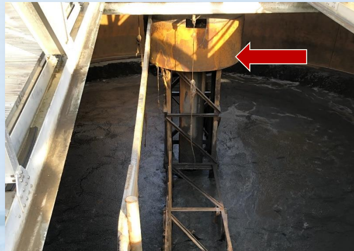
Repair Corrosion (Gravity Thickeners)
