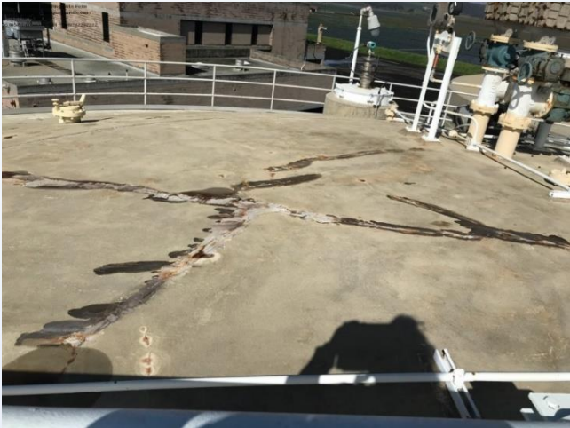
Repair Roof Cracks From Above (#2)
