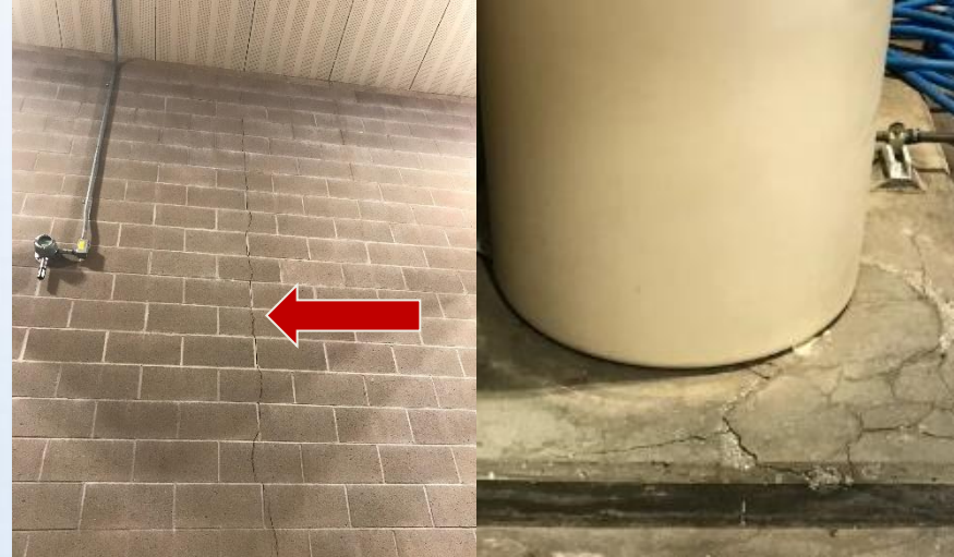
Repair Cracks/Spalling (Energy Recovery)
