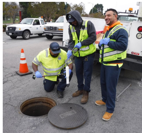
Mobile flow sensors are prepared to be lowered into the sewer system.
