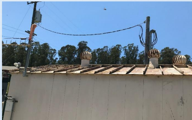
Recoat Corroded Metal Surfaces
