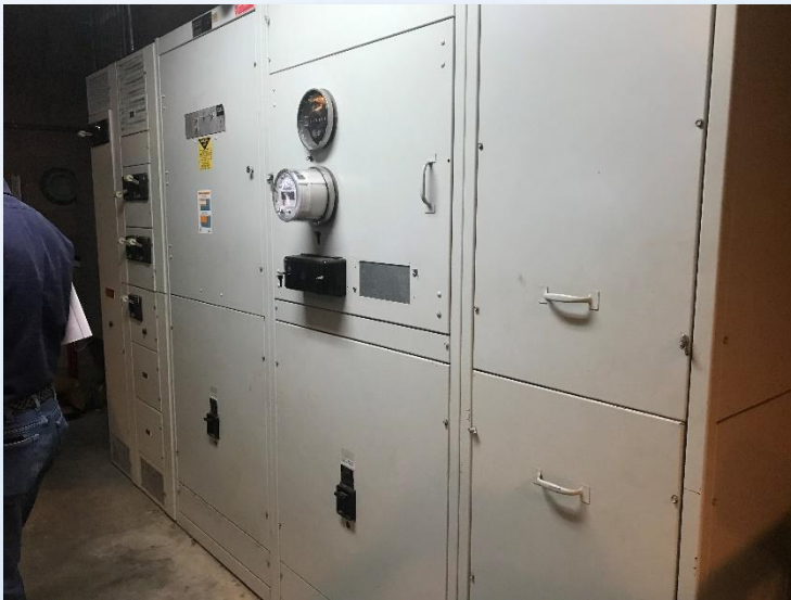
Electrical and Instrumentation upgrades needed due to end of useful life
