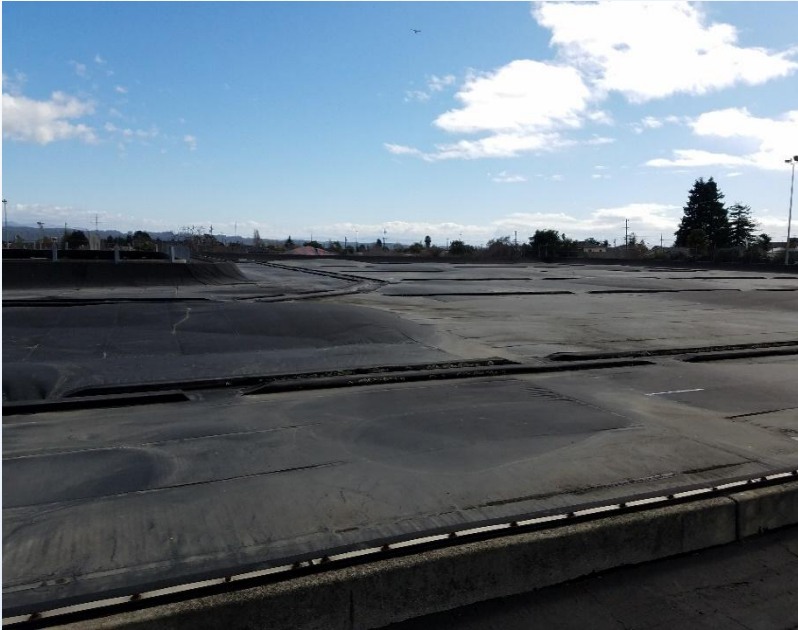
Freedom Reservoirs with Floating Covers (0.7 and 5.3 MG)
