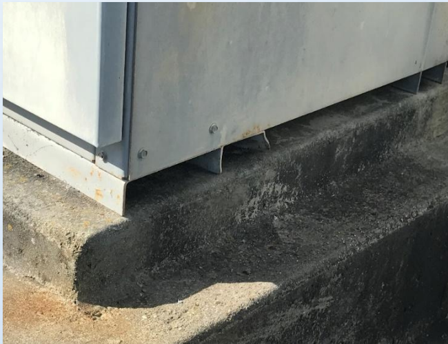
Electrical Panel Seismic Anchors
