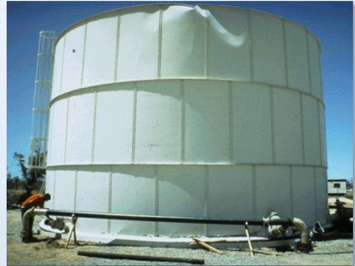
Example of Potential Seismic Damage
