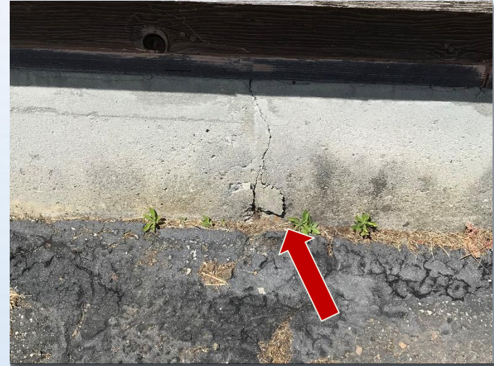
Repair Cracks or Spalling
