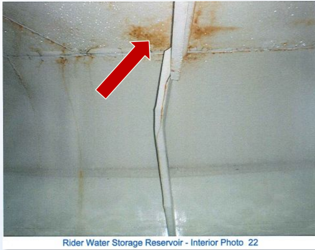
Tank Interior Corrosion (Four Steel Tanks)
