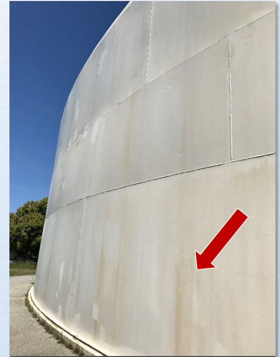
Tank Exterior Corrosion (Airport Tank)
