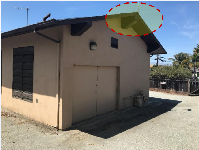
Anchorage of Roof Beams to Walls
