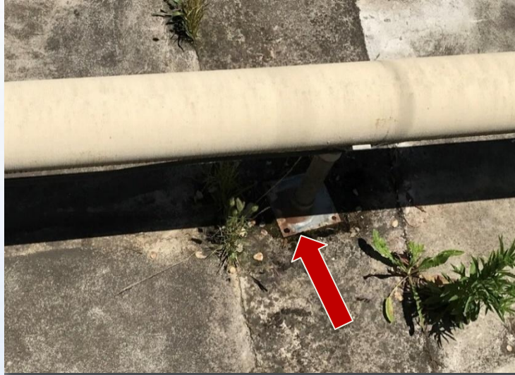
Replace Anchor Bolts at Pipe Supports
