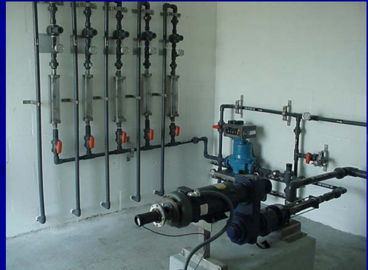
Alum Injection Equipment
