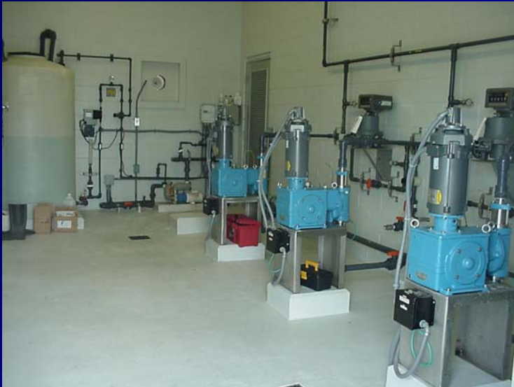
Alum Injection Equipment
