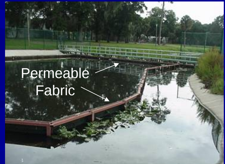
In-line Floc Trap
