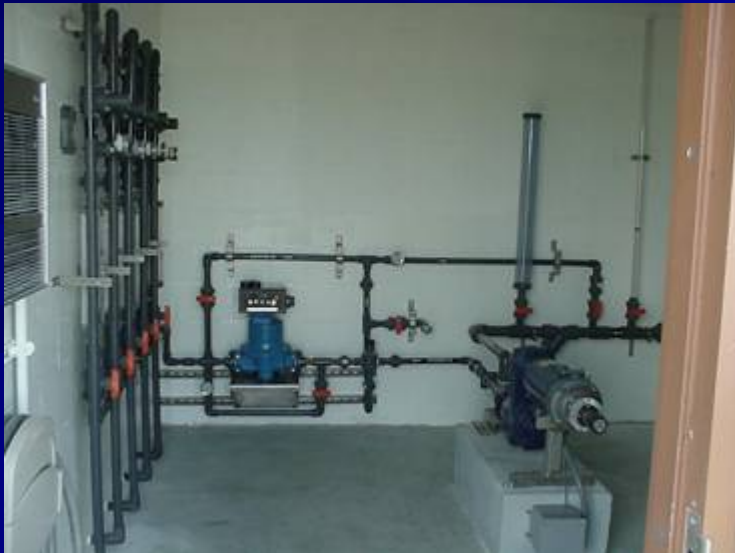
Alum Injection Equipment
