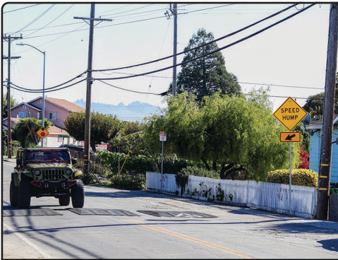
New speed bumps were installed on Roache Rd as a result of a Neighborhood Traffic Group Request.
