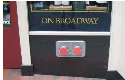
Example of an appropriately placed double standpipe connection in the base of a building at the sidewalk.
