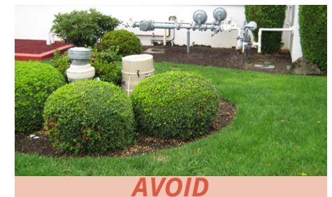
Example of inappropriately placed check valves and other utility devices in the front yard of a commercial building.
