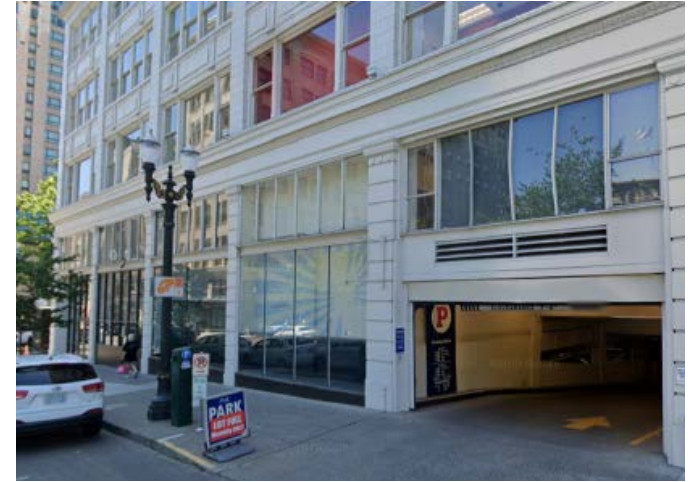
This parking structure is designed like a typical Downtown Building, and any ground floor parking is set behind commercial space with shopfronts lining the street. This building could easily accommodate other uses—such as
