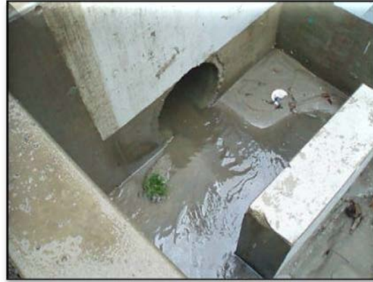
Treatment BMP Showing Sediment Pass Through
