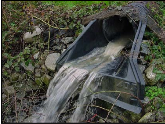
Treatment BMP Showing Turbid Discharge
